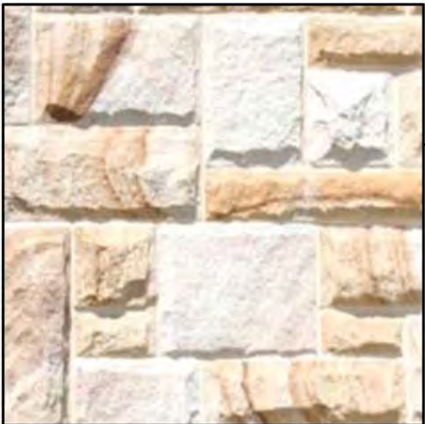
Sandstone basement walls
